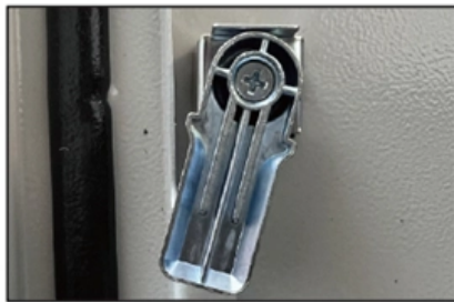
Strengthen door locks
