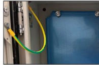
Grounding screw More aesthetically pleasing and safer
