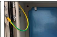
Grounding screw More aesthetically pleasing and safer
