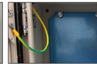
Grounding screw More aesthetically pleasing and safer
