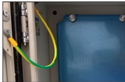
Grounding screw More aesthetically pleasing and safer
