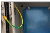
Grounding screw More aesthetically pleasing and safer
